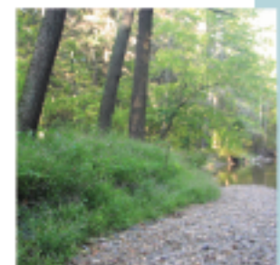
A state Growing Greener grant to the Conservancy was used to correct severe stream bank erosion in Jacobsburg Park.
