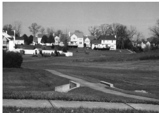
Drainage swale and recreation path, Hanover Township.
