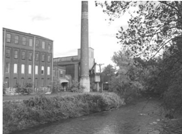
The Simon Silk Mill presents an opportunity to redevelop an abandoned industrial site into a business center for recreation-based enterprises as well as other economically viable ventures.
