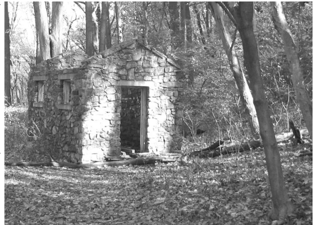
An example of a historic element that could receive an interpretive display.
