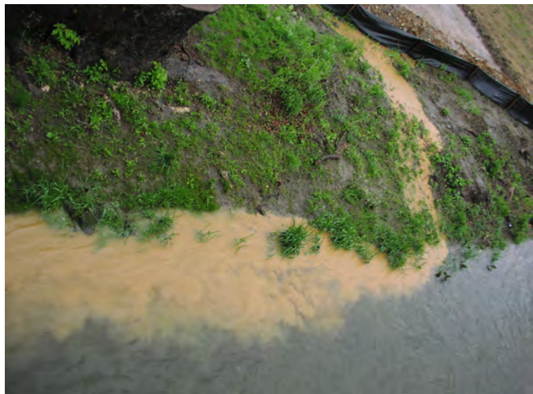
Sediment-laden stormwater runoff through an improperly installed silt fence
