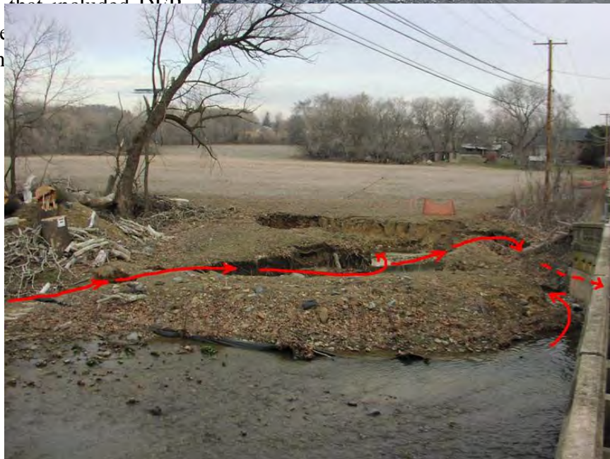
Sinkholes near Route 33 bridge Red lines depict direction of groundwater flow
