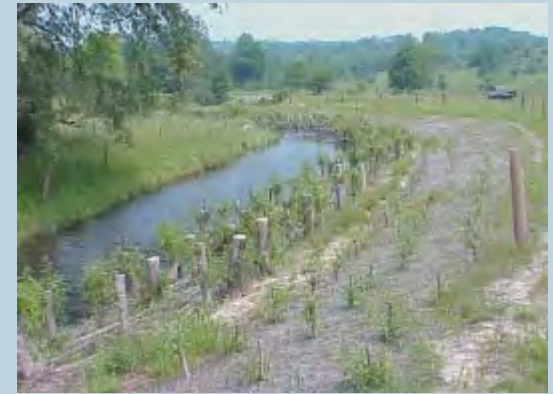
Photo of a newly constructed stream restoration area. In time, the live willow and dogwood cuttings and posts will naturally stabilize the streambank and restore the riparian area.
