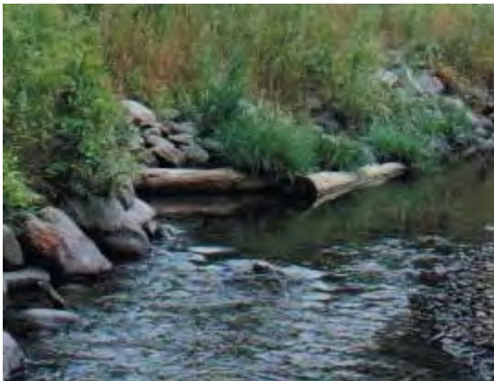
Stabilized streambank with fish habitat enhancement structures
